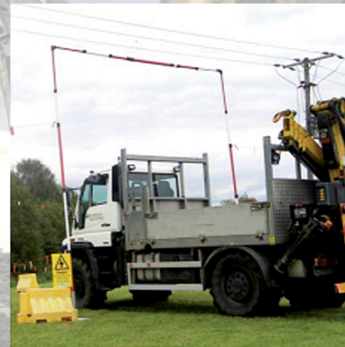
OVERHEAD ELECTRICAL LINES
